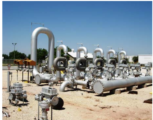
Micro Motion meters at pipeline gathering station
