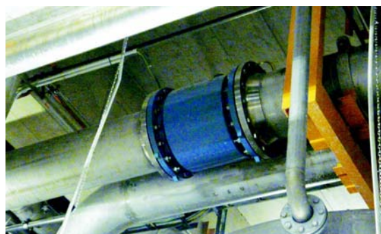
Rosemount 8700 magnetic flowmeter installed
