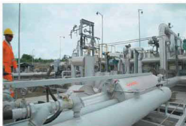
Figure 5. Each metering station has its own proving skid so that flow proving can be done in-situ at any time desired by Cairn or its customers.
