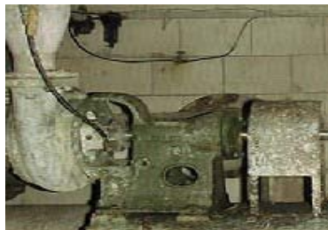
Cooling Pump for Boiler Feed Pump
