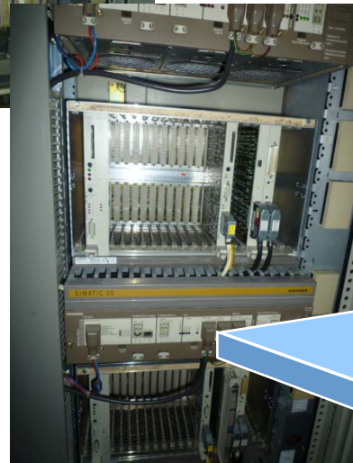
Obsolete Teleperm Controller and IO system
