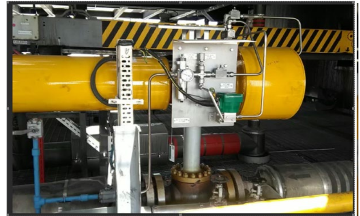
Installed AEV 2XC Ball valve
