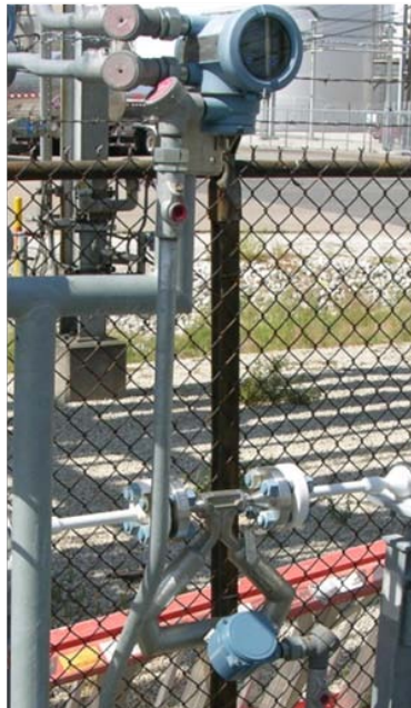
Ethylene custody transfer meter with Smart Meter Verification significantly reduces risk of lost production.
