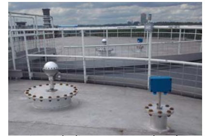
PRO parabolic antenna and multi-spot temperature sensor
