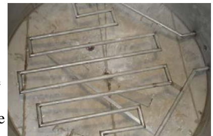
Heating coils near to tank bottom
